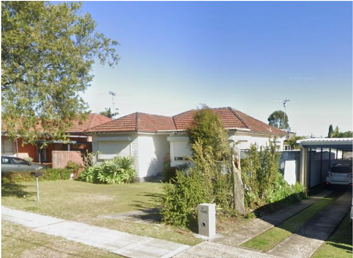
Figure 6 – Shows the neighbouring building at 18 Kiora st
