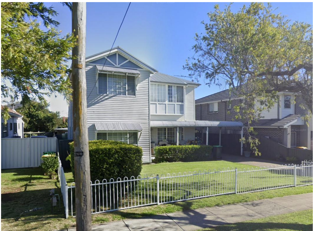
Figure 7 – Shows the neighbouring building at 14 Kiora st.
